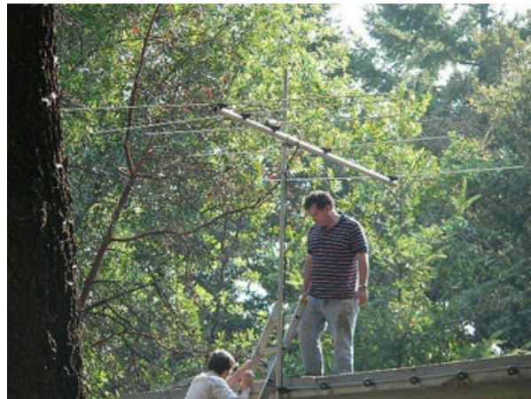
David Ritchie, W6DR, works to set-up the six-meter beam for the VHF/UHF station during a previous Field Day.
